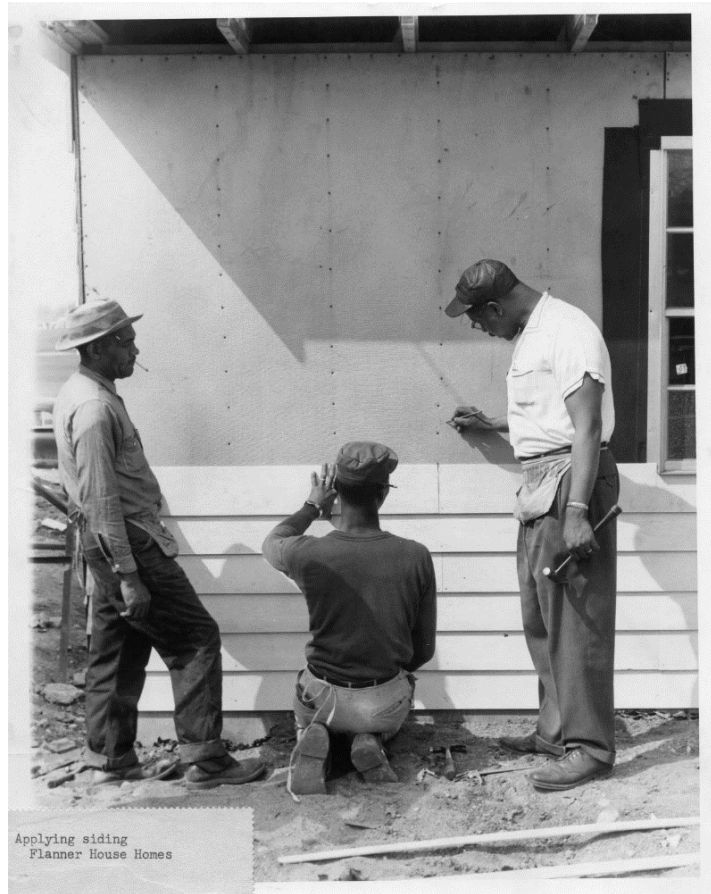
Carpenters applying siding to a Flanner House Home (Ruth Lilly Special Collections and Archives, IUPUI University Library, Flanner House (Indianapolis, Ind.) Records, 1936-1990 )
